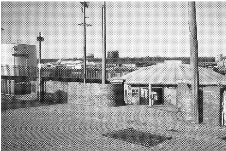
Entrance to Pedestrian and Cycle Tunnel viewed from the South.
